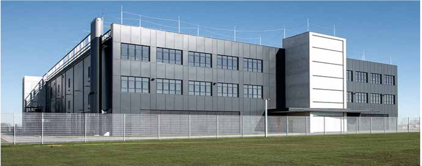
Amsterdam 1 Data Center
